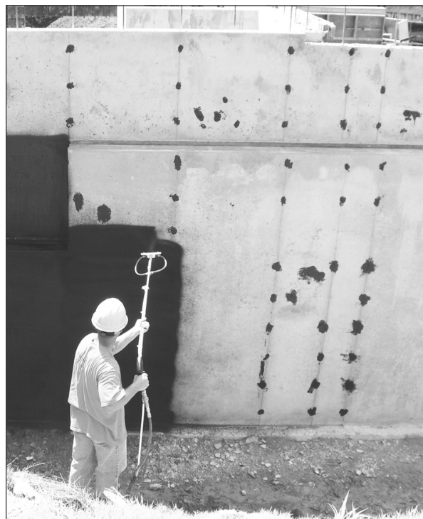
FIGURE 3 - SPRAY-APPLIED DAMPPROOFING TO FOUNDATION WALL
