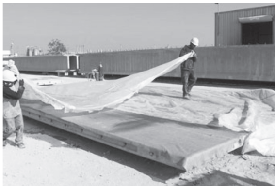
FIGURE 10 Burlap and Plastic Curing
